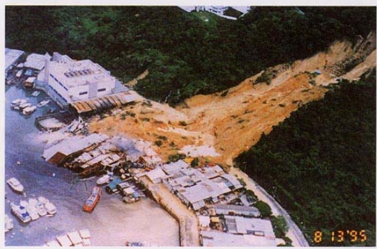
Fig. 1 The landslide above Shum Wan Road on August 13,1995
