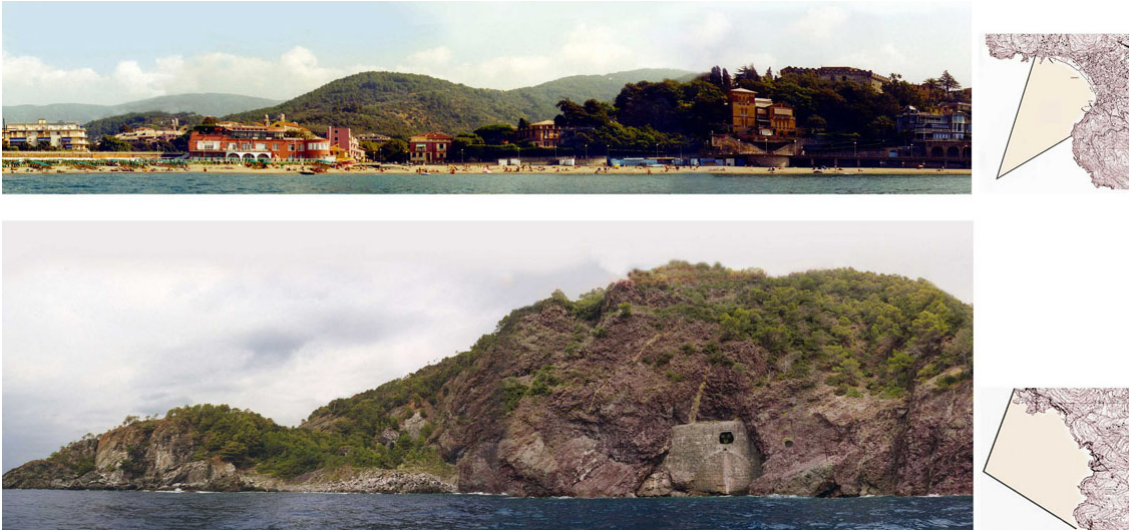
Fig. 6 Sea Front Map: particular of gulf of Levanto and old railway tunnel to support sea access system and cycle tracks
